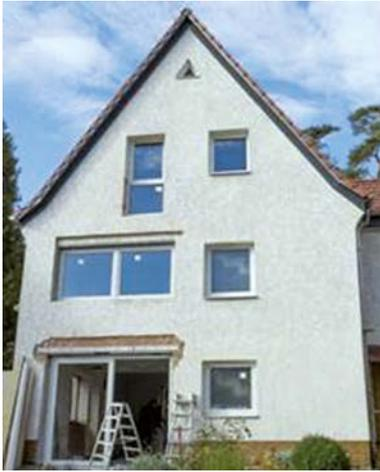
Fig. 1. Element newly installed during refurbishment with fall-protection glazing (window in top floor left) with enlargement of the window areas
