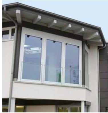
Fig. 2. “Window handrail” for protection against falling, mounted on a window frame
